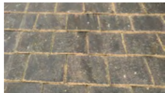
Slate / stone roof
