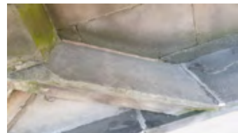
Lime Mortar - pointing
