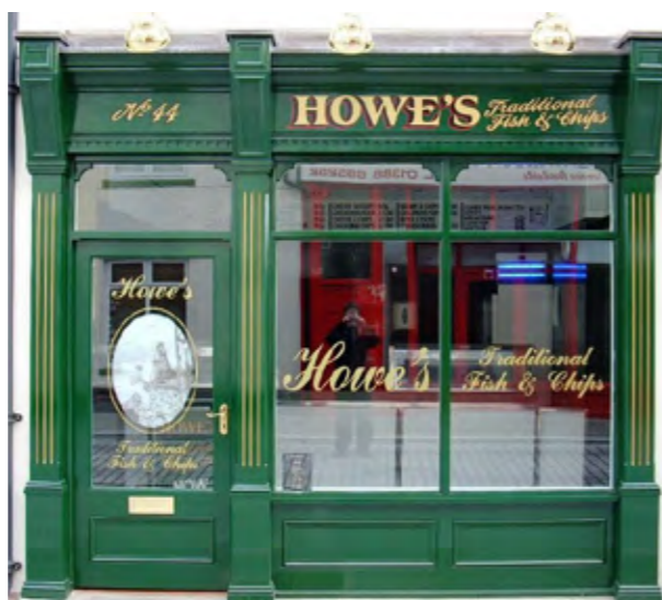
Well maintained shop front
